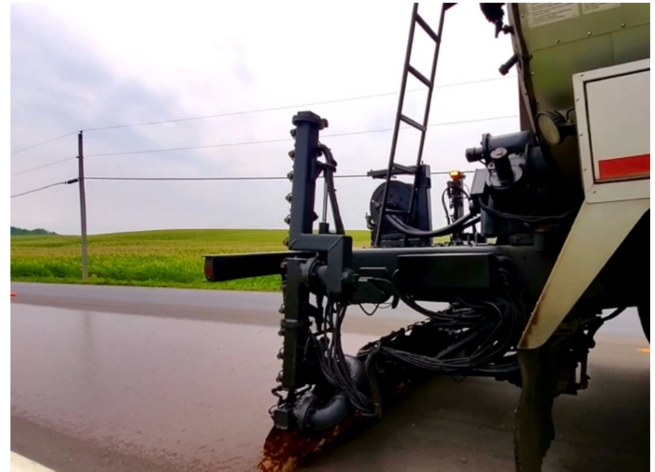
Application of SOR on an asphalt pavement
